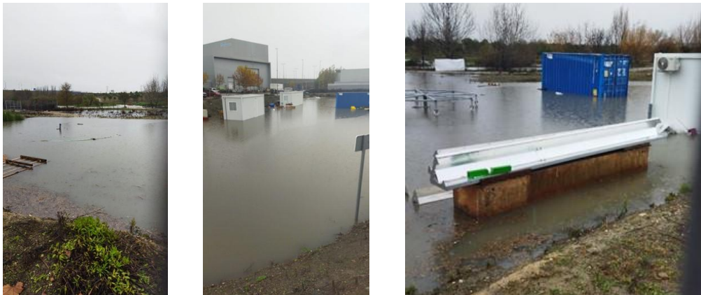
Fig. 7. Images of the test site during the flooding.
